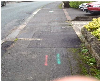
Photos showing condition 3 footway – Functionally Impaired
