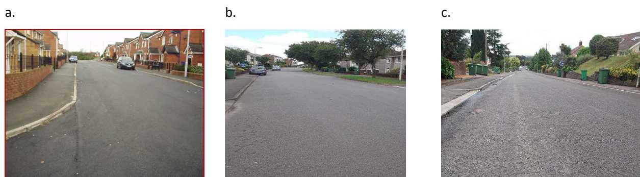
Photos illustrating a range of green condition roads that require no treatment
