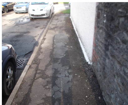
Photos showing condition 2 footway – Aesthetically Impaired
