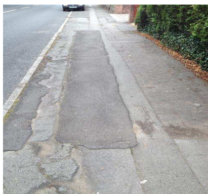
Photos showing condition 4 footway – Structurally unsound
