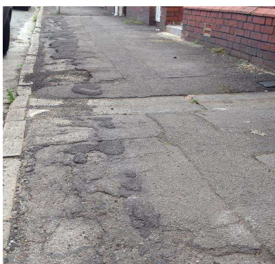
Photos showing condition 4 footway – Structurally unsound
