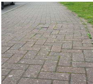
Photos showing condition 2 footway – Aesthetically Impaired
